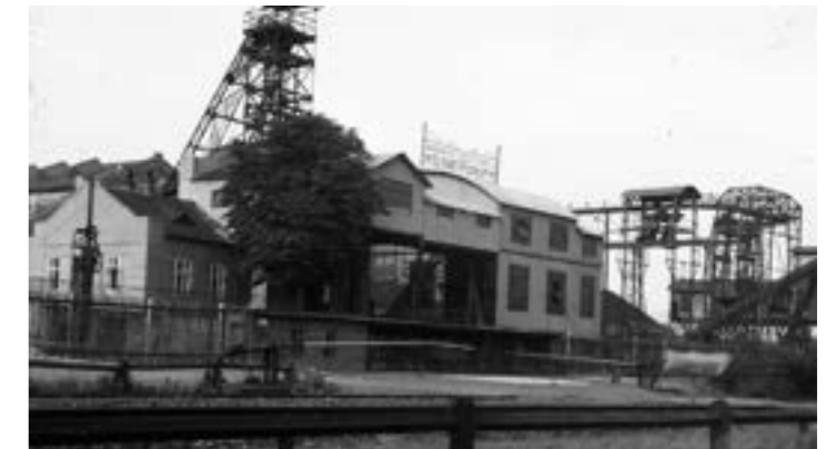
Trmice, šachta Elizabeth, 1900
